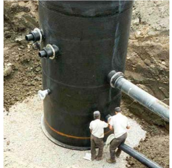
FIGURE 3A: PLACE MANHOLE ON STABLE FOUNDATION
