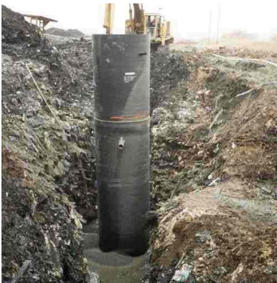
FIGURE 1B: MANHOLE TRENCH IN LANDFILL
