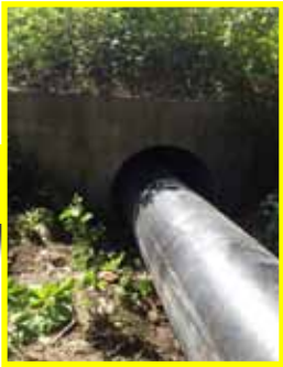
The first piece of Snap-Tite HDPE is lowered into position and inserted into the host pipe.
