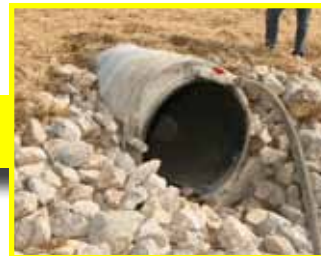
The grout is pumped into the entire length of the pipe, filling in all voids between the new and host pipe, and the areas between the pipe and roadway.
