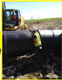
A gasket is installed on the next piece of pipe, assuring a watertight seal when connected, meeting ASTM D3212 requirements.
