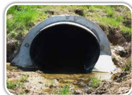
A culvert, rehabilitated with Snap-Tite® oval pipe.
