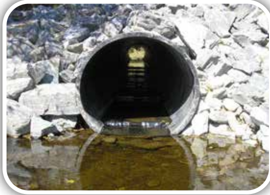
Pools adjacent to culvert can play important design elements in ISCO A.L.P.
