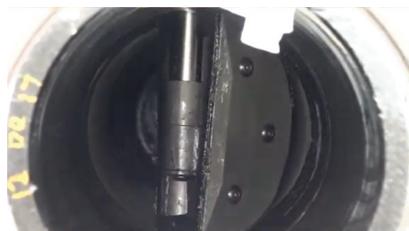
Folded plugging head is inserted into pipe vertically, through a hot-tapped hole.
