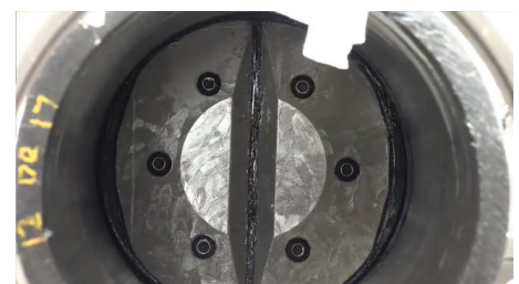
Opened plugging head is turned perpendicular to the main, like a butterfly valve, and the flow of product is stopped.
