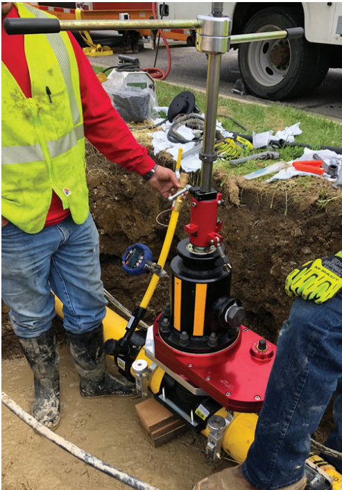
Permanent repair with electrofusion fittings following an emergency squeeze-off.
