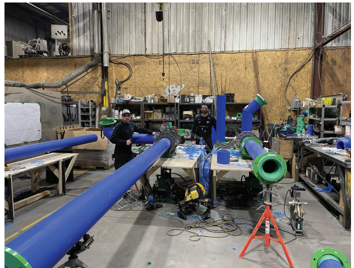
Pre-Fabrication of Main Line Spools in Shop
