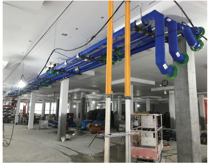
Installation of Main Lines on Site
