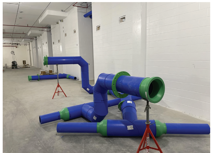
Pre-Fabricated Main Line Spools
