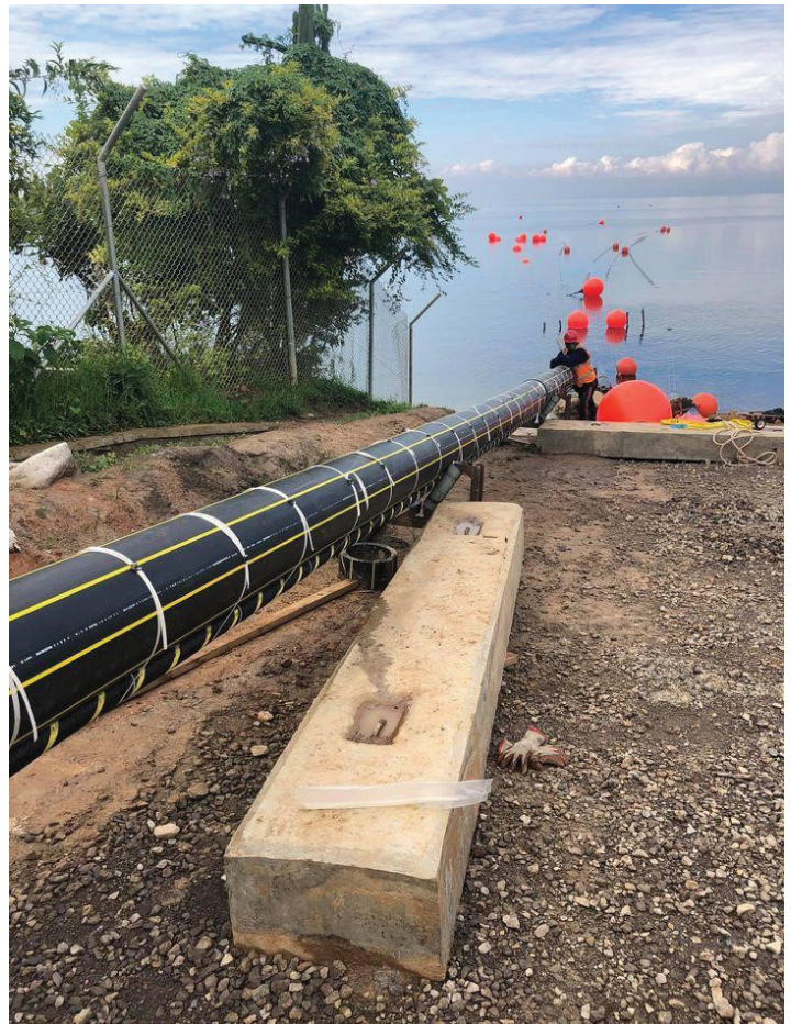
Above: The 12" HDPE submerged export pipeline carries methane gas from the barges in Lake Kivu to the onshore power plant. Below: A 1400mm (55") manifold was included within the raw water riser. It is used to initiate flow and carry water to the gas-water separator.
