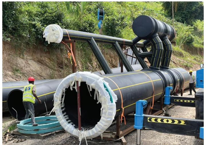
Above: The 12" HDPE submerged export pipeline carries methane gas from the barges in Lake Kivu to the onshore power plant. Below: A 1400mm (55") manifold was included within the raw water riser. It is used to initiate flow and carry water to the gas-water separator.
