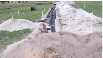
of golf irrigation pipe system failure results from water hammer. When exposed to water hammer, breaks and leaks occur at the weakest points of conventional pipe systems, the joints. A system made up of HDPE pipe is more durable and can withstand surges in water pressure. HDPE pipe's flexibility allows it to bend to a radius 25 times its diameter, meaning fewer 90 degree bends overall. The flexibility lessens the chance for water hammer to damage the pipe and also lessens the chance for leaks.
