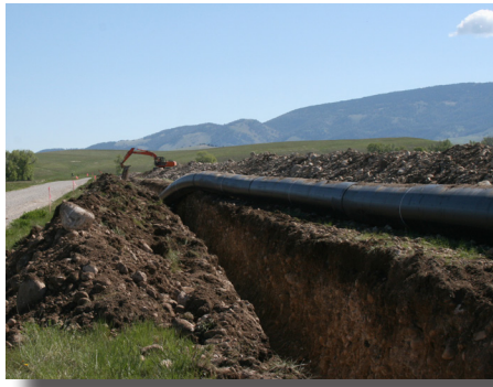
Large-diameter HDPE pipe is placed underground.
