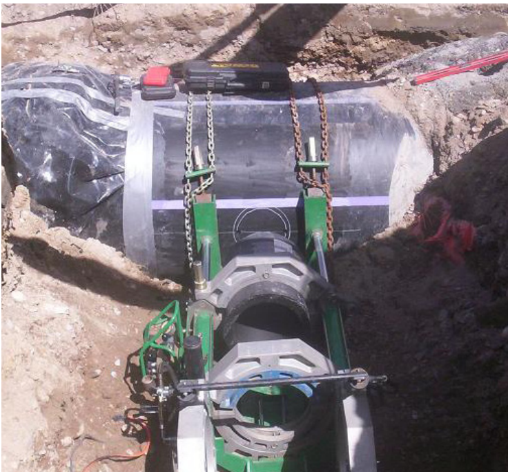
Side fittings are fused to the large-diameter pipe.
