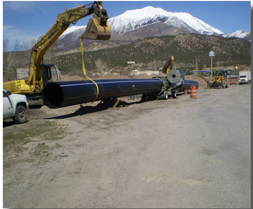
Large-diameter pipe being brought on site and fused.
