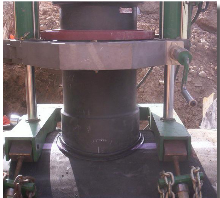
Side fittings are fused to the large-diameter pipe.
