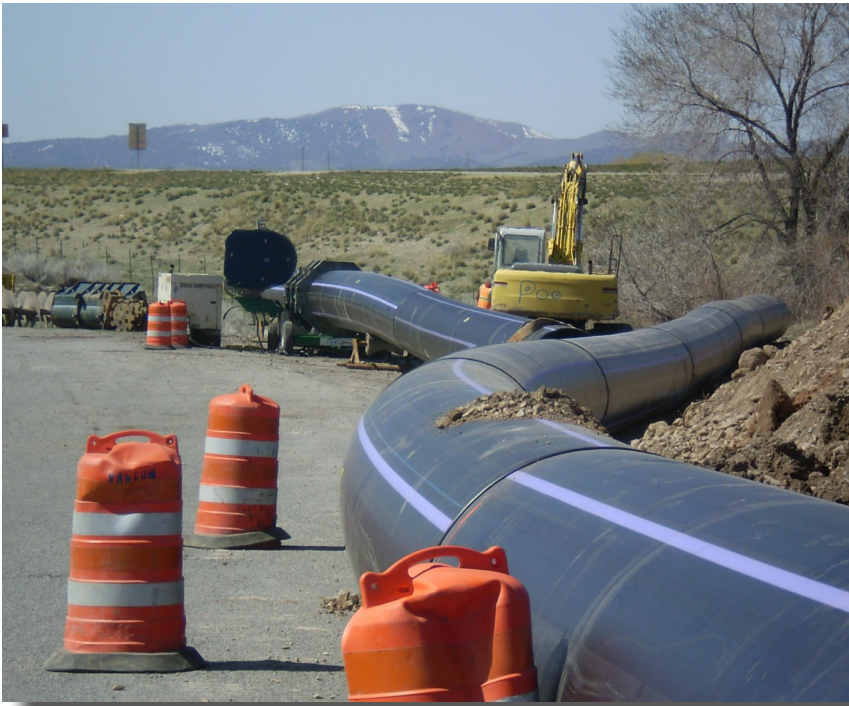
The flexible HDPE large-diameter pipe snakes around corners and rugged terrain.
