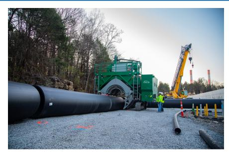
HDPE pipe, which involves less heavy equipment and manpower needed for the job.
