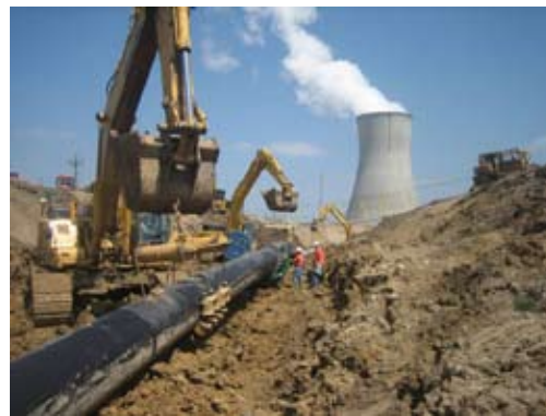
Installation of the 36-inch DR 17 HDPE cooling tower blow down line.
